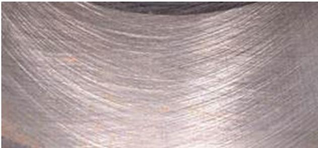
Fig.139: New honing profile and crosshatching with the right angle
